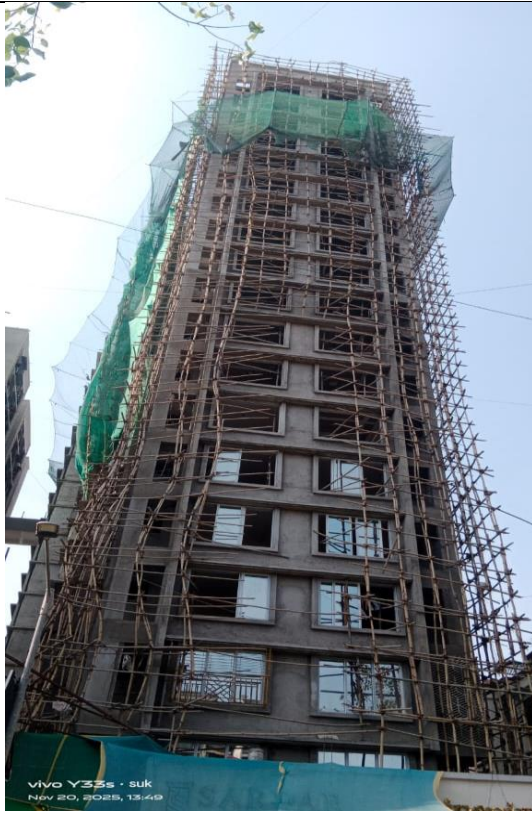
Rehab Wing D, E
