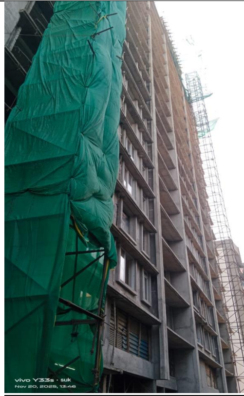
Rehab Wing D, E
